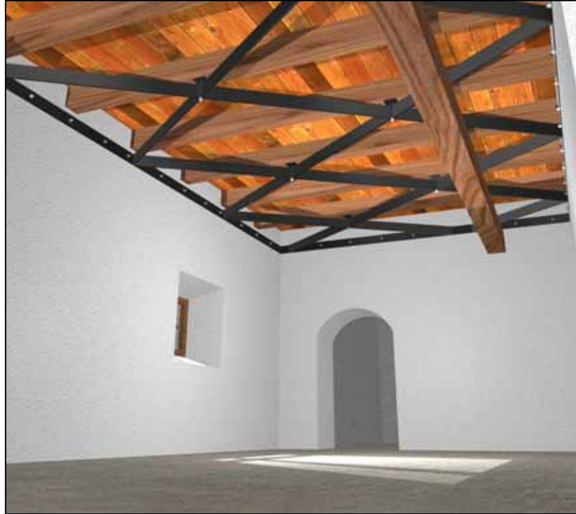
FIG.2: The spatial steel structure under the first floor
