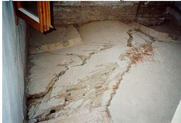
Figure 9. “Cristo” church in Rovigo – structural damage to the vaults.
