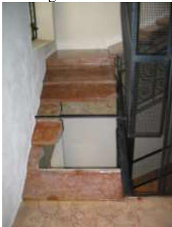
Figure 12. Stair collapse in a masonry building in Milan
